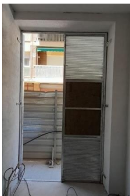
Interior puerta CT
